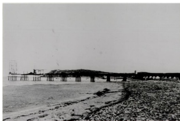
Barwon Heads Bridge under construction 1927
